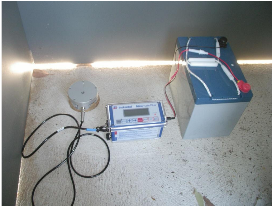
Plate 1 Instantel Minimate Plus and geophone (typical arrangement within a secure shed)
