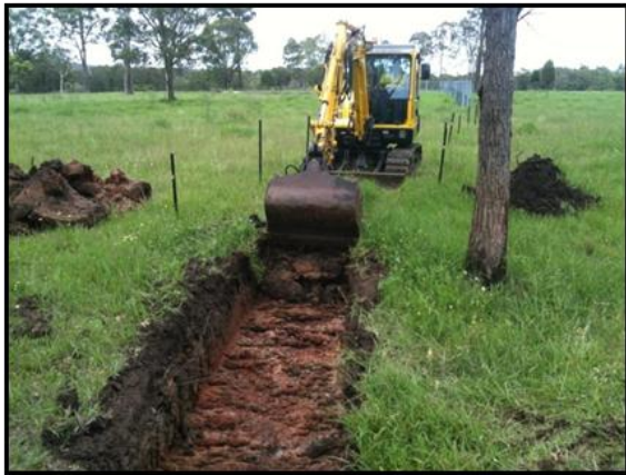
1. Excavator digs to remediate surface cracking
