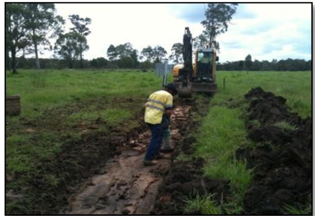
2. Area compacted and re filled
